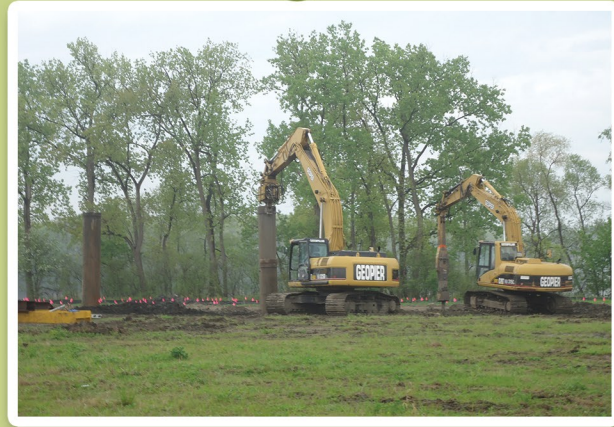
The digging begins, Spring 2014
