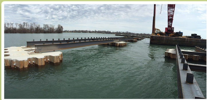
3.30.2016 Reaching 700' into the channel of the Detroit River
