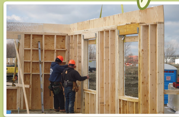
2015 The walls go up!
