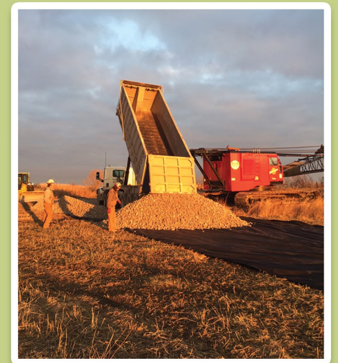
12.17.15 Pouring Aggregate Preparation for the fishing pier begins
