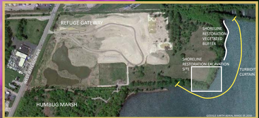
Google Earth Aerial Image • 05.2010
