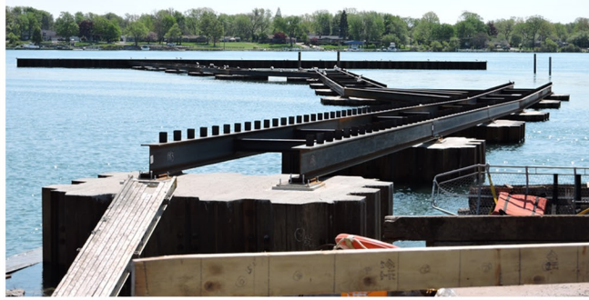
Fishing pier and school ship dock construction is 70% complete! Photo: FWS
