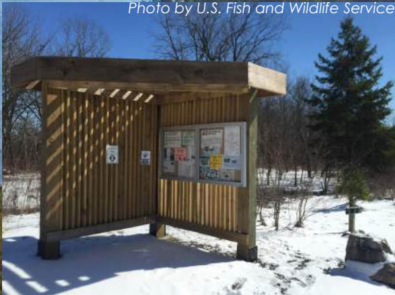
A new kiosk at Gibraltar Bay Unit.
