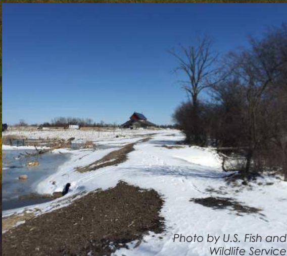
Infrastructure upgrades at the Monguagon wetland allow for better flood protection and water level control.
