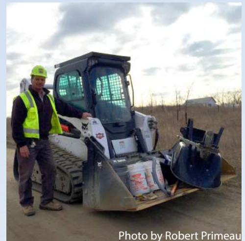
Photo by Robert Primeau Refuge maintenance mechanic John Nicely poses with the Bobcat track loader after completing construction work at the Refuge Gateway.
